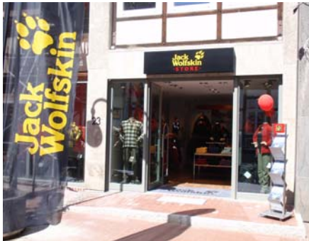
Bäckerstraße, Goslar (after renovation)
