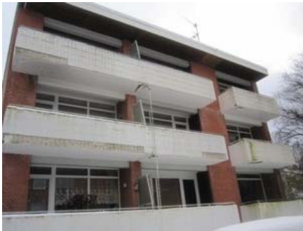
Cloppenburger Straße, Oldenburg Balconies before renovation
